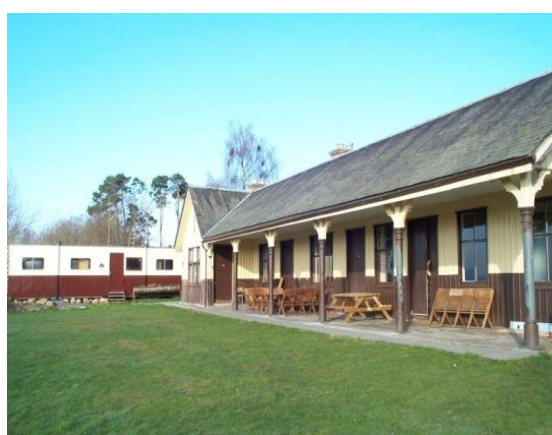
The day services centre at Redcastle Station
